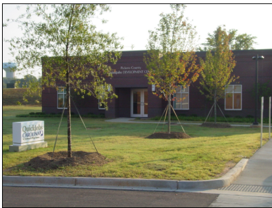
Pickens County QuickJobs Development Center
