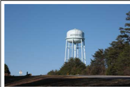
ACOG worked with the City of Westminster to secure funding to upgrade their water treatment facility and construct a new 500,000-gallon elevated storage tank.
