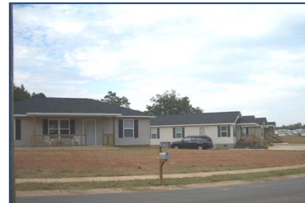
ACOG is providing administrative support for the CDBG-funded Hope Acres Habitat for Humanity Project in Gaffney.
