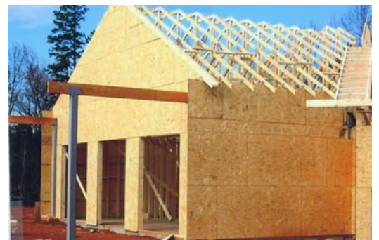
Construction is underway on the new Cowpens Senior Center, which will house a host of activities and programs for the senior population living in Cowpens and the surrounding vicinity.
