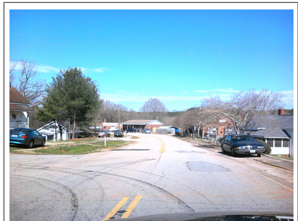
The Catechee Mill Village in Pickens County will receive grant funds for construction of almost 2,500 feet of water lines.
