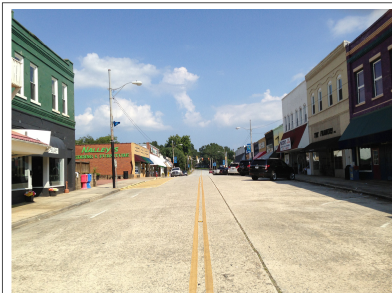
CDBG funds will be used for a number of infrastructure improvements along Commerce Street in downtown Liberty.
