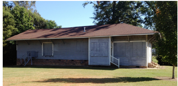
Williamston will be renovating the historic depot into a farmers market.
