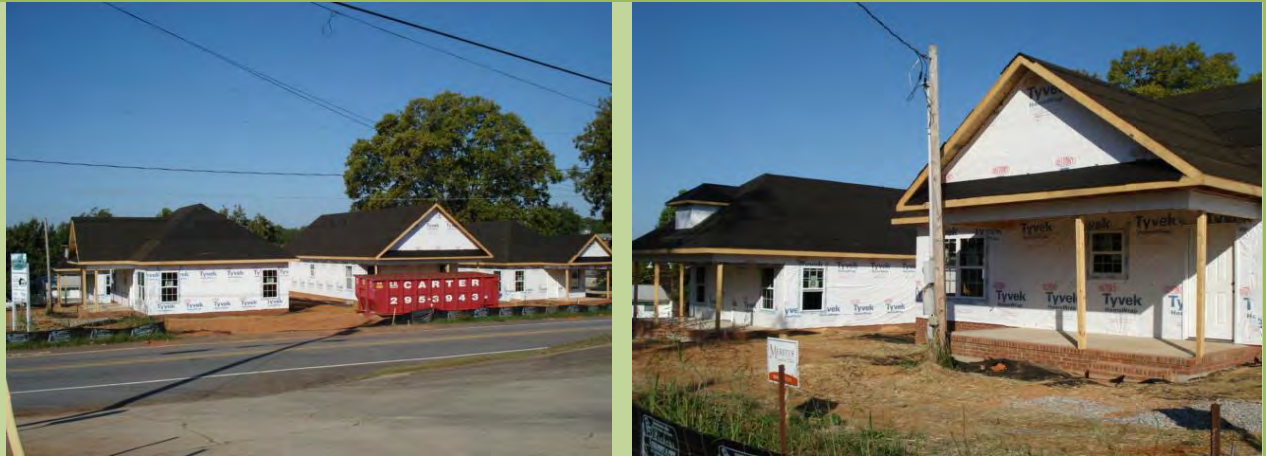
The photos above of the four LMI houses under construction at 312 S. Lewis Street were taken in September of 2011. Completion is anticipated before the end of 2011.
