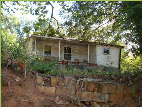
One of many vacant houses in the Study Area.
