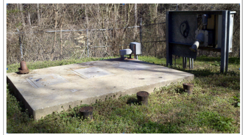
Cavins Road Pump Station
